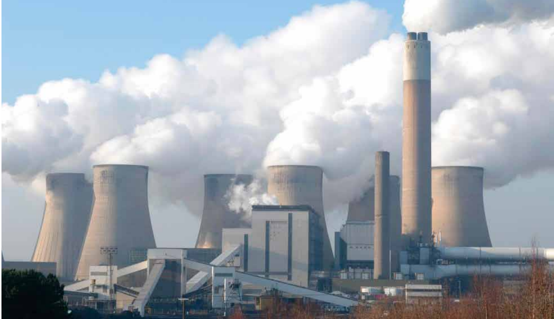
Ratcliffe-on-Soar coal-fired power station (2000 MW) and FGD plant (in foreground).
