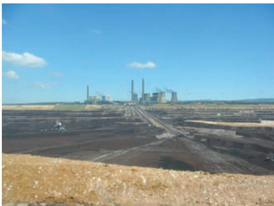
CO 2 capture and storage (CCS) is the only the way to achieve near zero emissions from coal-burning power plants, such as these in the Latrobe Valley, Australia.
