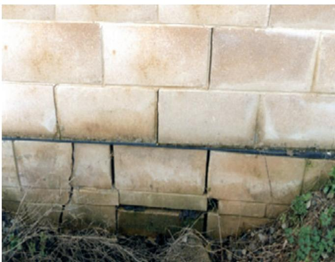
*Severe heave, in Fuller's Earth (montmorillonite) under a squash court at Monkton Combe, Bath. The heave is caused by the expansion of the clay minerals as they absorb water.*
