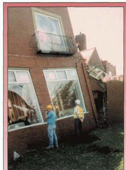
*Holbeck Hall Hotel, Scarborough, destroyed when the adjacent cliffs suffered a rotational landslide.*
