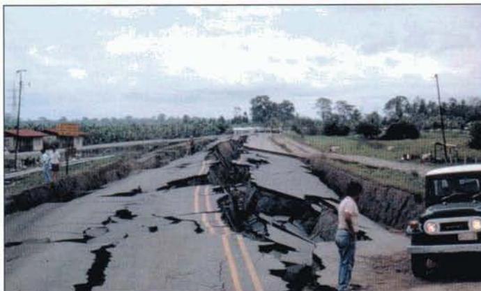
Lateral spreading of road embankment at Cuba Creek near Limón, Costa Rica, caused when the ground below liquefied during the April 22nd, 1991 earthquake.
