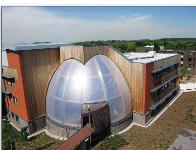
Views from the tower crane of the William Smith Building construction.
