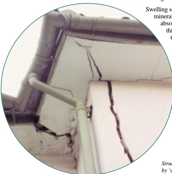
*Structural damage caused by 'centre lift'.*
