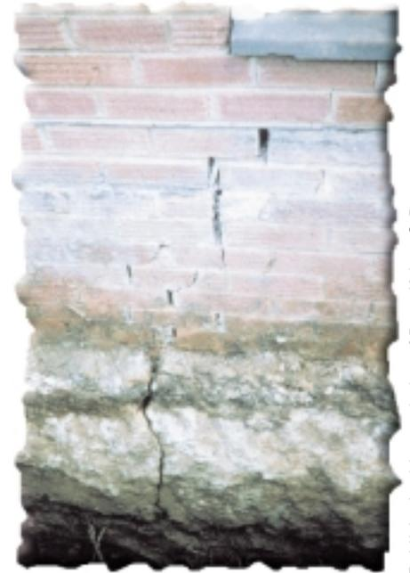
*Structural failure caused by 'end lift'.*
