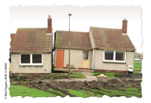
Ferniehill Terrace, Gilmerton. A bungalow and its raft foundation rotated by the subsidence of mineworkings in the Gilmerton Limestone, 2000.
