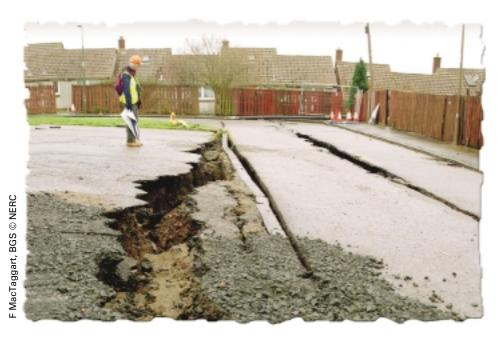
Ferniehill Street, Gilmerton. Open fissures near the southern limit of the subsidence of mineworkings in the Gilmerton Limestone, 2000.
