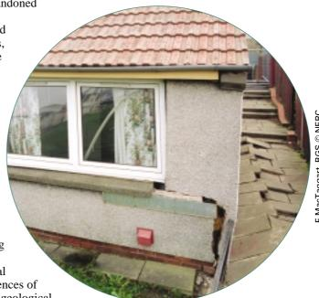
Ferniehill Street, Gilmerton. Compressive damage caused by the subsidence of mineworkings in the Gilmerton Limestone,
