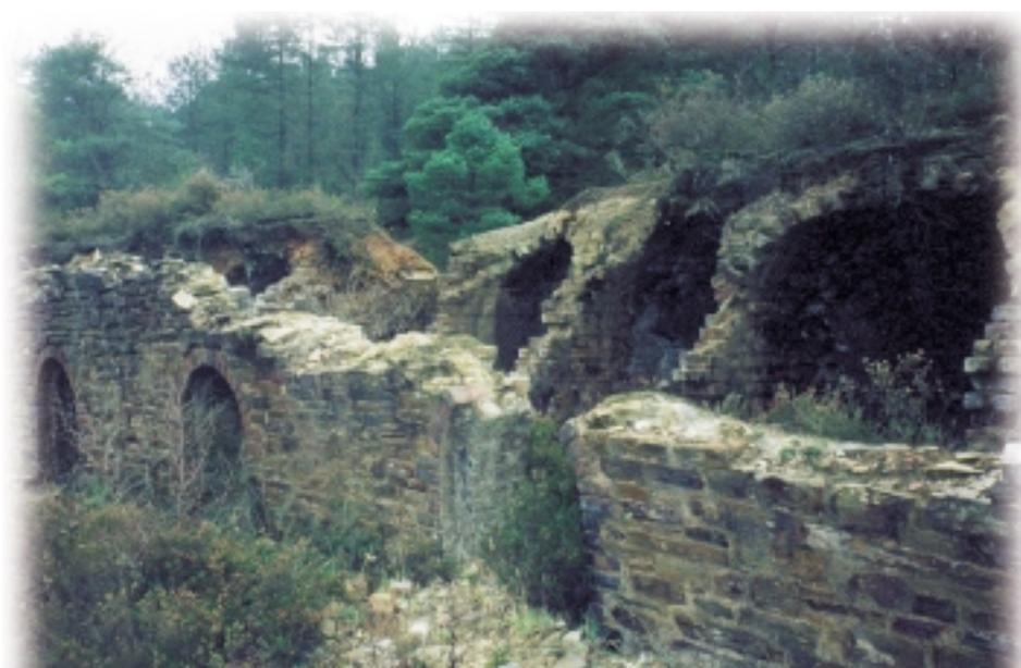
Derelict Brunton arsenic condenser at Devon Great Consoles mine. Arsenic oxide was previously produced at the works by roasting arsenopyrite. Elevated levels of arsenic were found in soil samples taken at the site.
