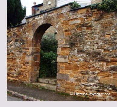
In older buildings the ironstone has crumbled and deteriorated. Lower levels in the succession were known as the "Bastard Stone" by quarrymen as it contained no iron ore. At Lyddington (below image), the English Heritage property "Bede House" built in the late 15C is an good example of a building using Northampton Stone with Limestone quoins and decoration, also used in the Braunston cottages, with smaller blockwork being prevalent.
