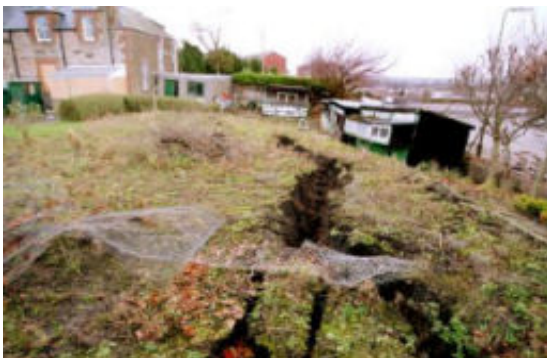
The affects of mine subsidence, Edinburgh Photo Copyright: BGS©NERC
