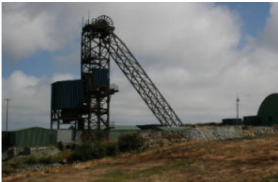
Parys Mountain shaft Photo Copyright: BGS©NERC
