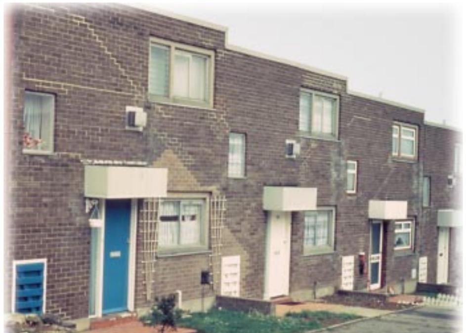
*Diagonal crack in new terrace due to swelling of London Clay along former hedge-line, Vange, south-west Essex.*
