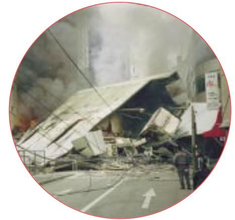
*Concrete frame office building completely destroyed in Kobe earthquake of 1995.*
