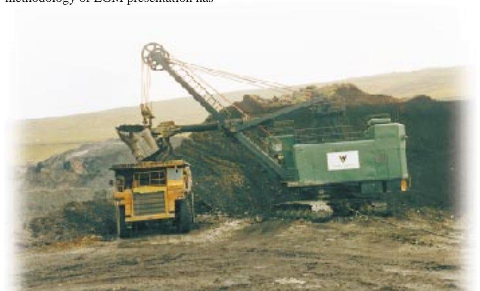
*The East Merthyr Reclamation Scheme in South Wales. The scheme involved the removal and safe disposal of iron smelting slag from a derelict industrial site above old shallow mine workings followed by an open-cast operation to recover coal from the pillars of the abandoned shallow workings and to extract additional coal from below the old workings. Finally, the site was infilled, landscaped and restored to a condition suitable for housing, other industrial or recreational use.*
