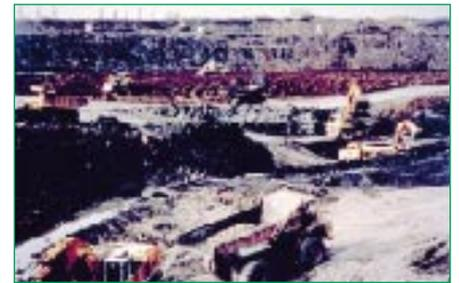
*Redevelopment of the Bowman's Harbour site near the centre of Wolverhampton involving excavation of the shallow coal deposits beneath old landfill.*
