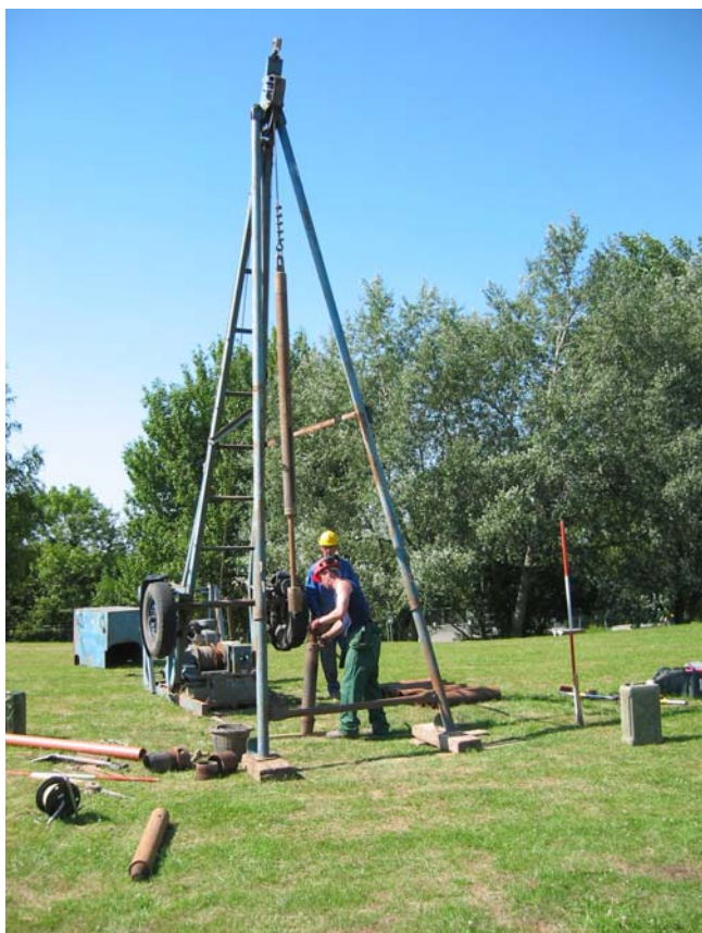
Shell and auger drilling
