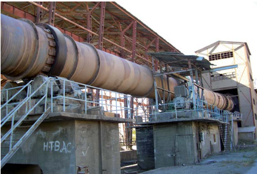
The Jebel Seraj Cement Enterprise in Parwan province, produces cement made using clinker purchased from Ghuri cement plant.
